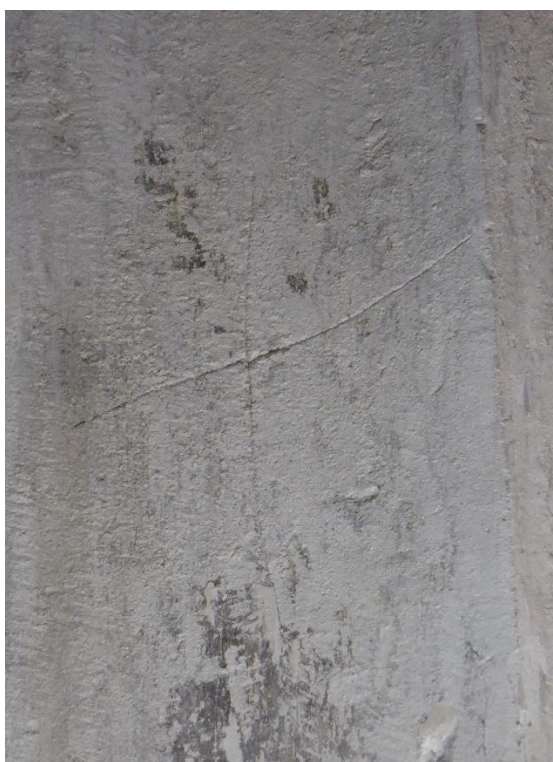
Fig 14 Chancel, north window, east side Cross, possible mason mark. Photo 136
