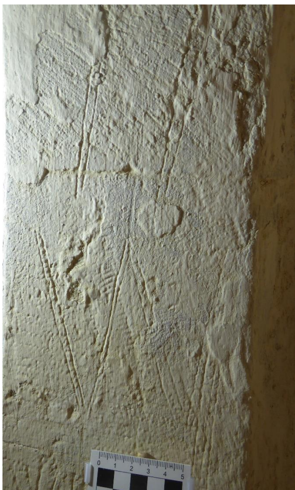
Fig 3 West doorway, south side. V shapes. Photo 112
